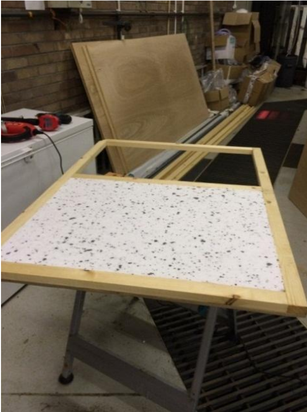
Above: Soundproof baffles under construction for the dumbbell tank.
