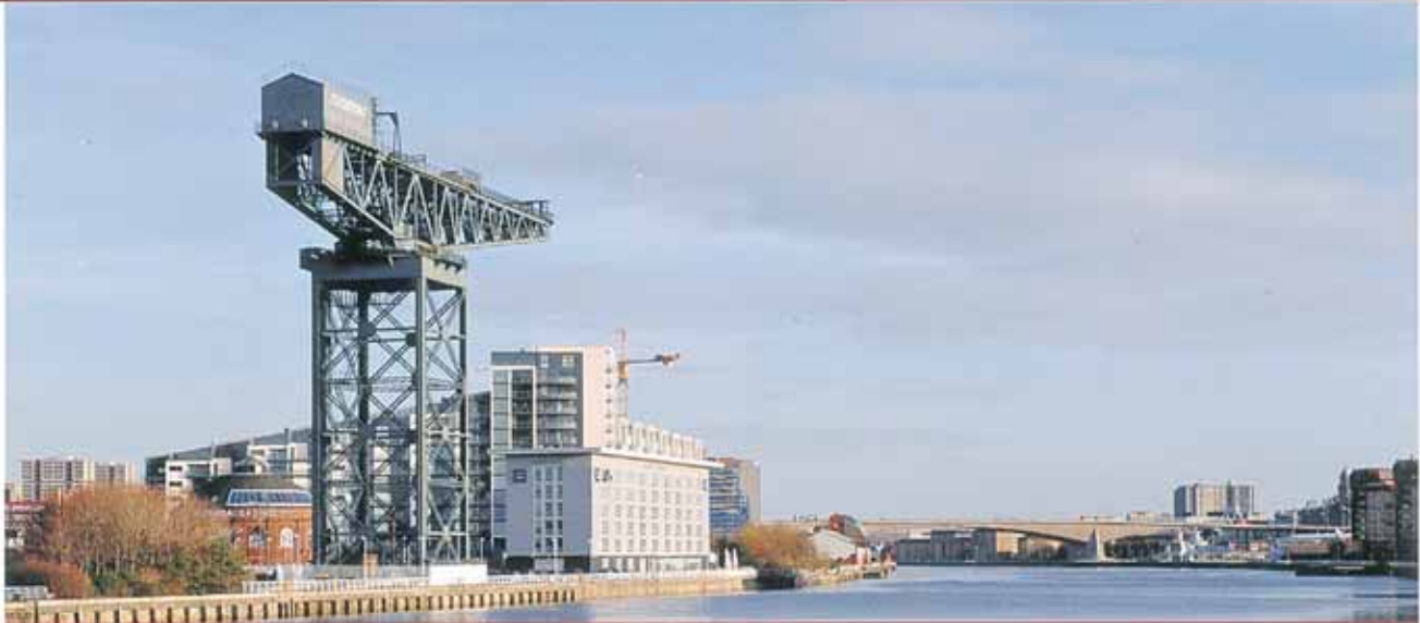
The Finnieston Crane on Stobcross Quay in Glasgow's docks, a 59 metre high cantilever crane built in 1932 to load heavy machinery onto freighters and transfer boilers and engines into new vessels
