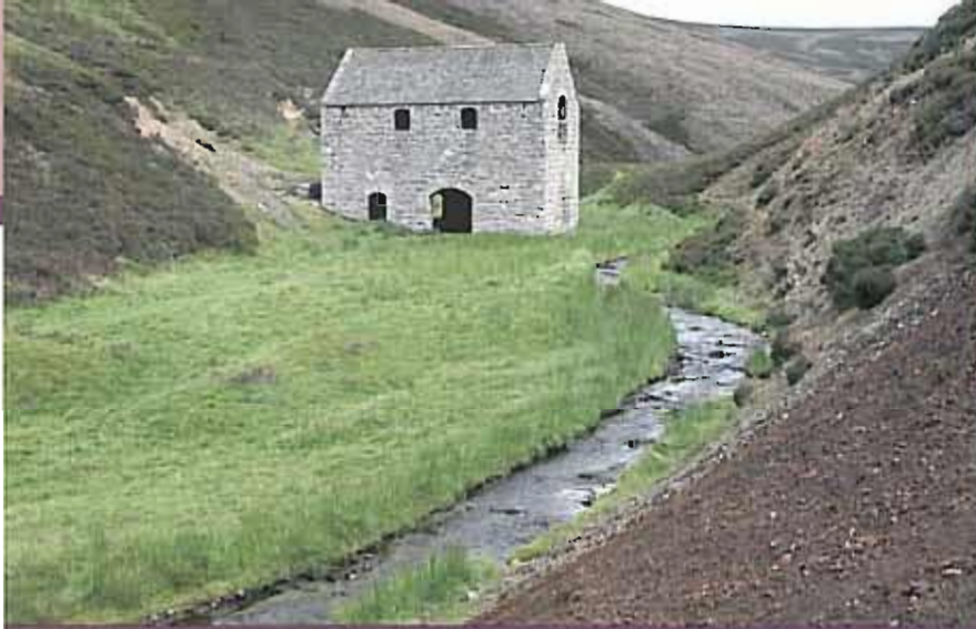
Old mine buildings at Lecht Mine near Well of the Lecht
